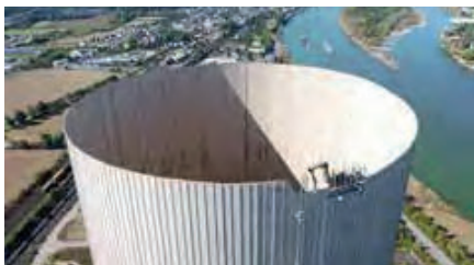
In total, some 3.790m 3 of material was dismantled during during 6 months.
